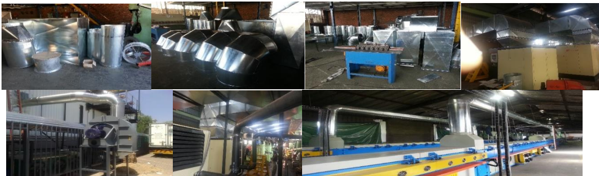
Factory extraction systems
